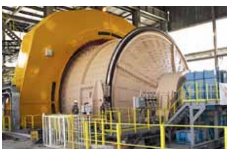
A typical zinc concentrator plant
