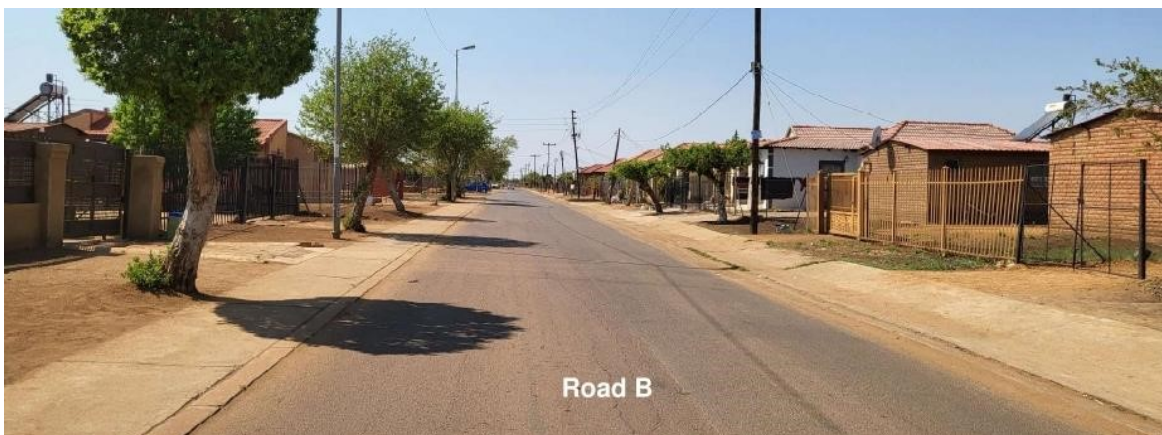
Figure 10: Existing Pedestrian Walkway along Road B (eastbound view along Road B)
