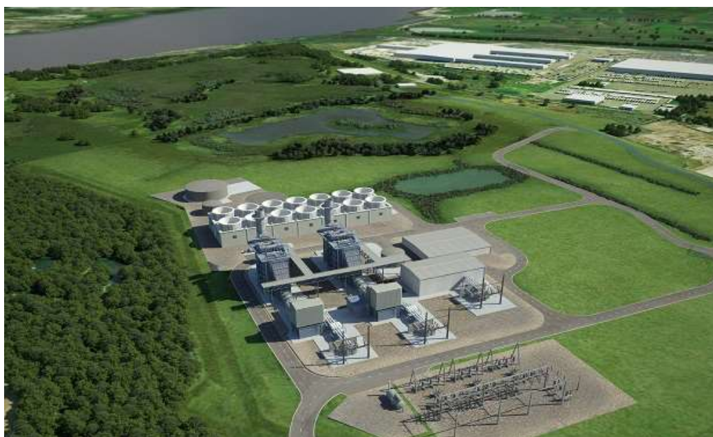
Figure 3.3: Aerial view of a typical gas to power plant
