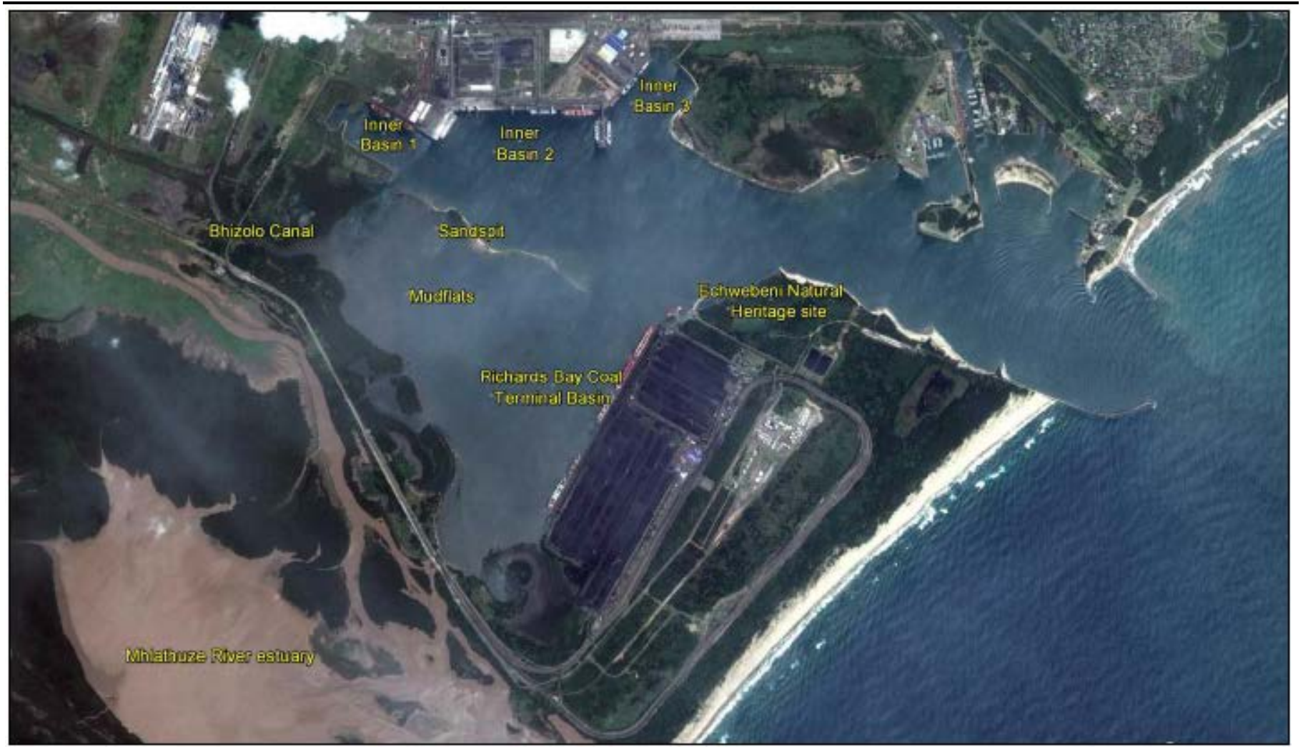
Figure 5.5 Map of Richards Bay showing the location of Inner Basin 1 where the FPP is proposed to be moored
