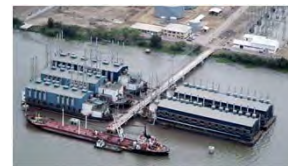
Bunker barge servicing multiple FPP
