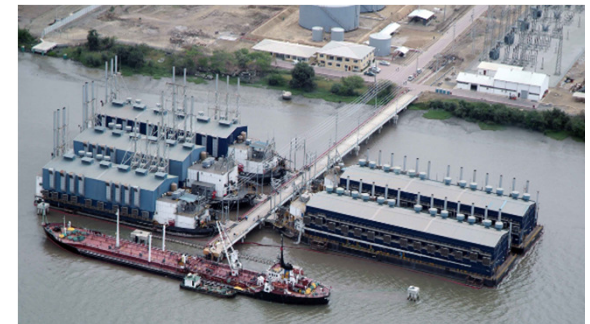
Bunker barge servicing multiple FPP
