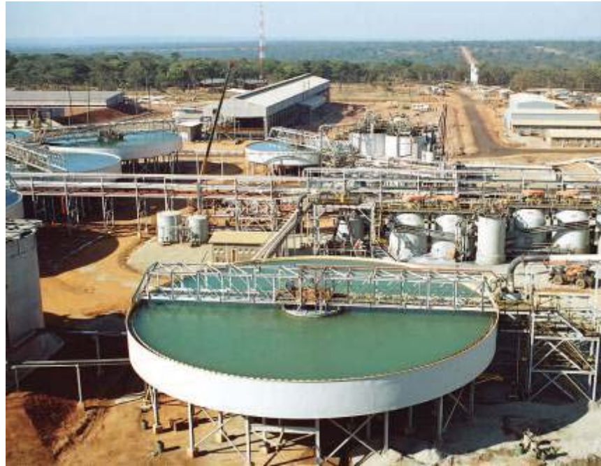
Figure 3.6 Typical image of concentrator plant
