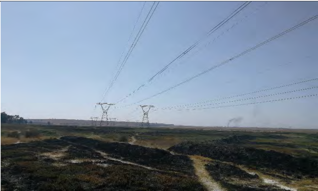
Powerlines near the Proposed Project Site. Just north of dump 7L5 and 7L6.
