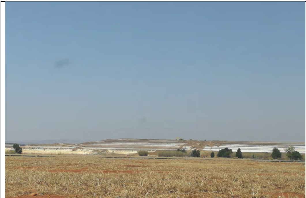
7L3 Zinc Tailings Storage Facility Reclamation Project, located approximately 1 km north-west from Site 1 of the Proposed Project site.
