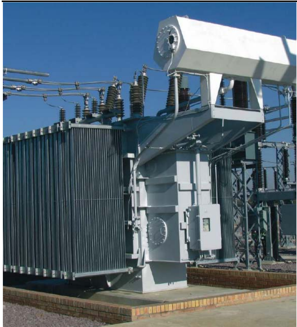
Figure 4.8 Power Transformer
