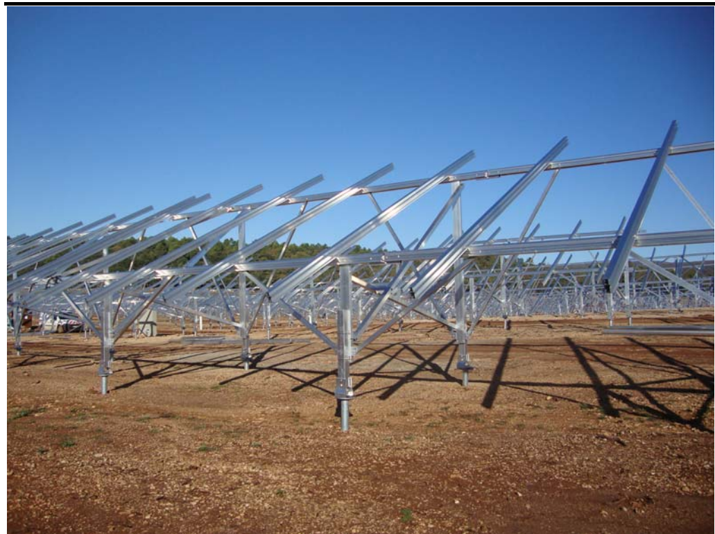
Figure 4.3 Typical Anodized Aluminium Frame
