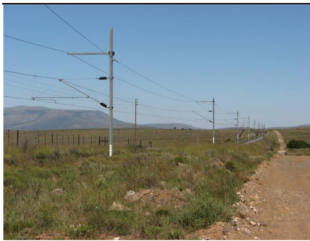
Figure 5.12 View of Site, Looking South, Showing Existing Railway Line
