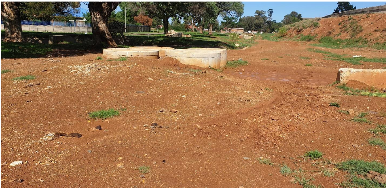
Figure 7: Disturbed area due to pipe construction
