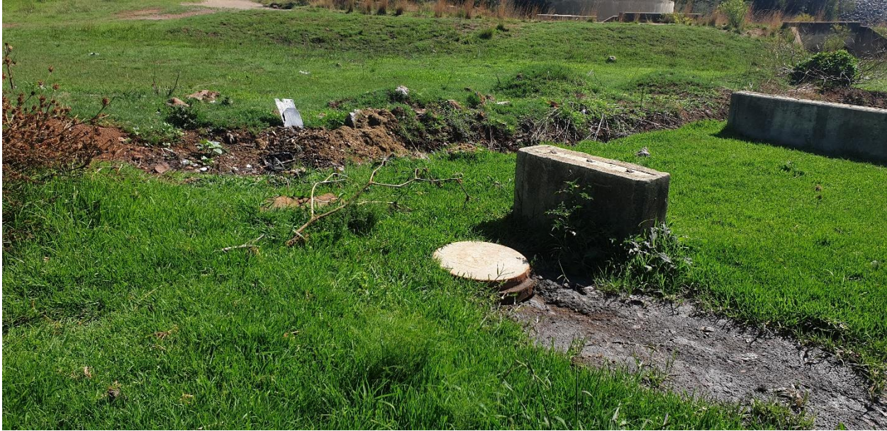
Figure 8: Sewer coming out of the pipe close to the site
