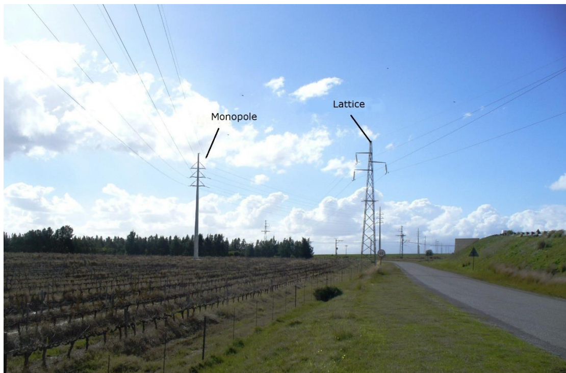
Figure 6: Typical 132 kV power line structures
