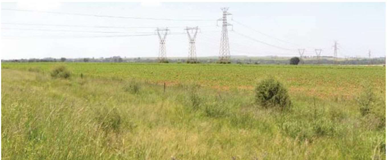
FIGURE 10: VIEW OF EXISTING POWERLINES LOCATED WITHIN THE STUDY AREA.
