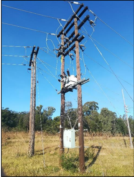
Images 4: Eskom NB1 11kV overhead feeder
