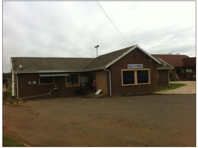
Photo 2: The existing Head of Works to be upgraded
