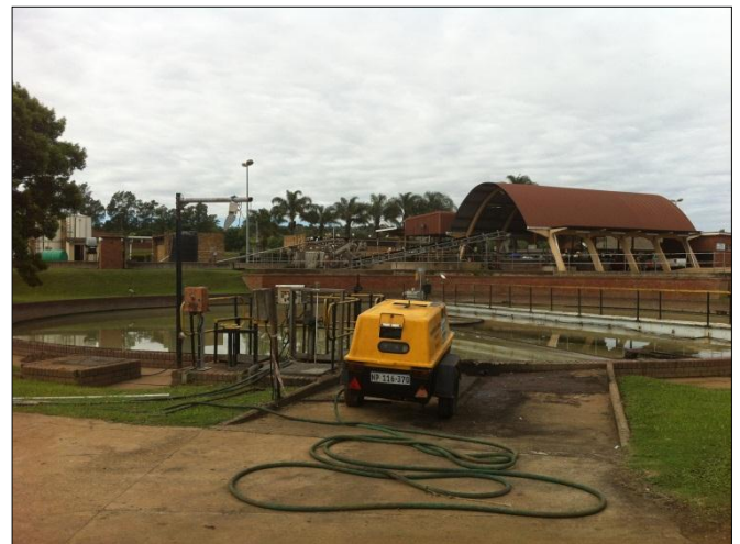
Photo 4: One of the two existing primary settlement tanks
