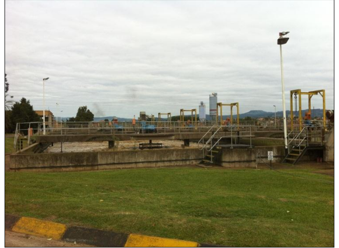
Photo 8: The existing aerobic reactor to be converted to an anaerobic reactor during the upgrade
