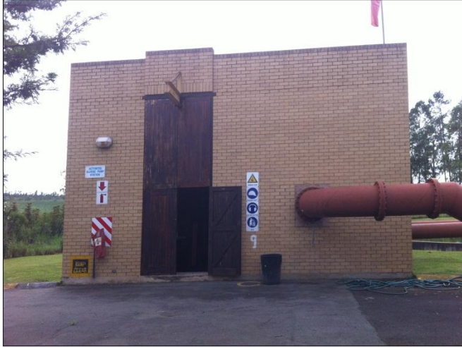
Photo 7: The existing activated sludge pump station
