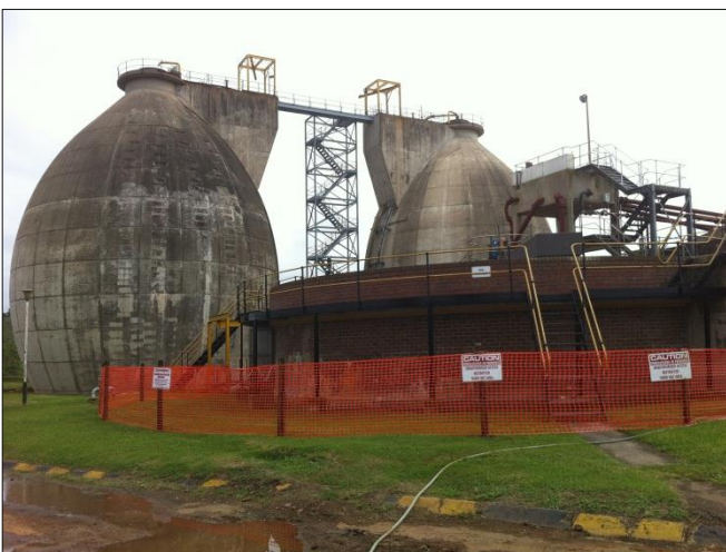
Photo 5: The existing two egg shaped digesters
