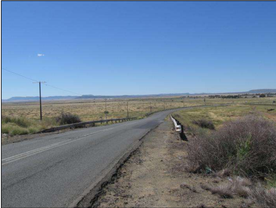
Figure 35: View from the R48 west of De Aar toward the application site
