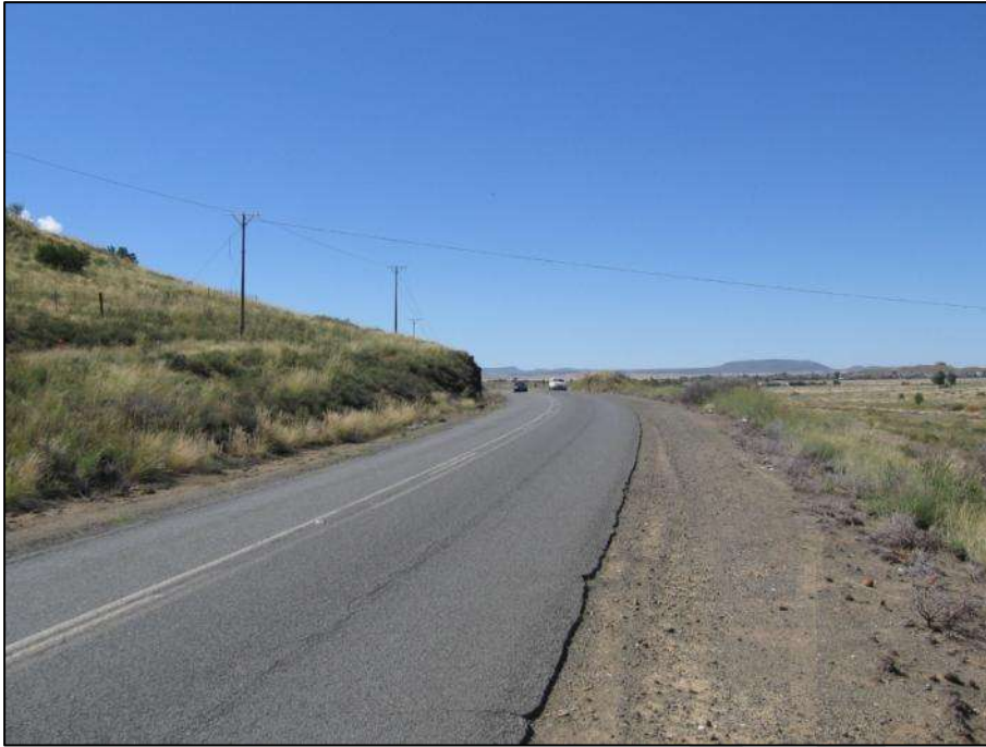
Figure 36: View from the R48 showing how hills to the west of the site will restrict views of the proposed solar energy facility
