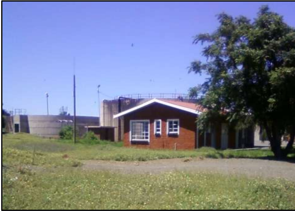
Figure 20: The De Aar Sewage Processing Works
