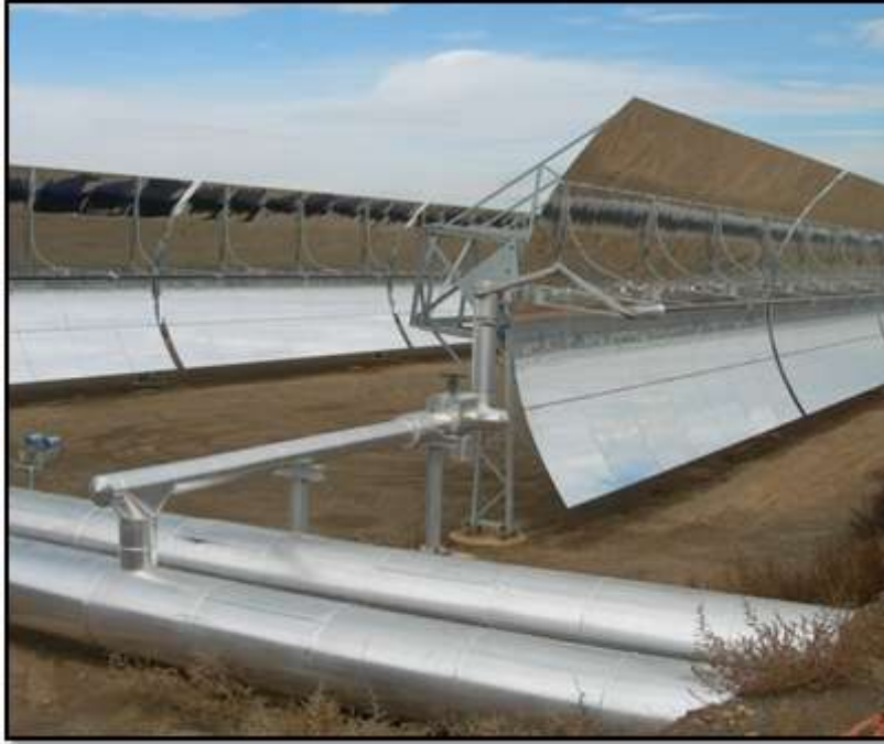
Figure 4: Parabolic trough solar collector assembly
