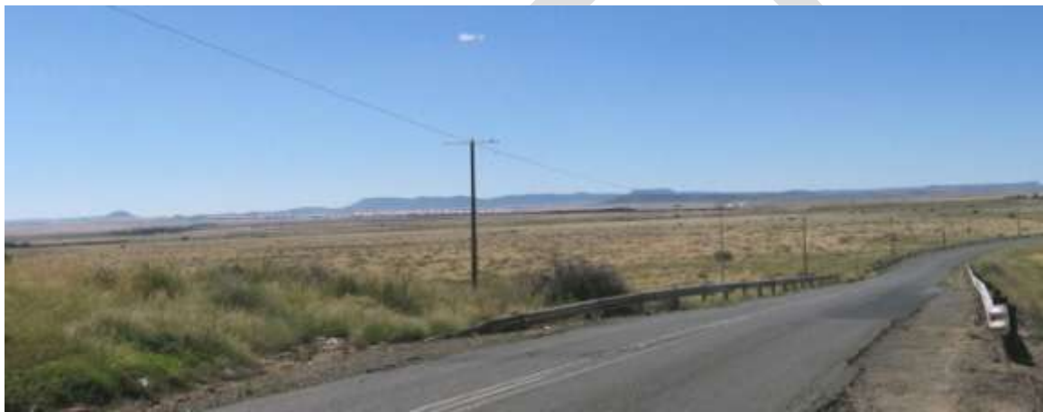
Figure 44: Visually modelled post construction panoramic view toward proposed solar energy facility from the R48
