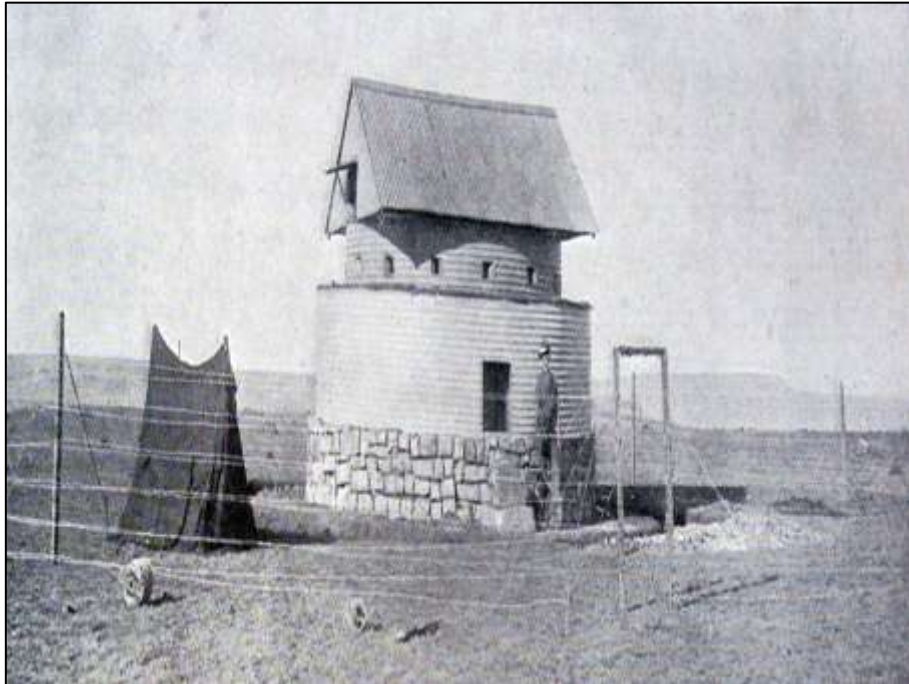
Figure 62: Rice pattern blockhouse with barbed wire fencing
