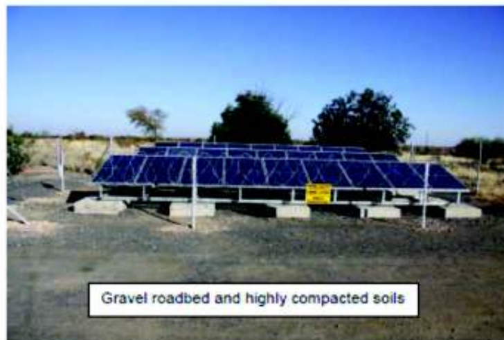
Figure 12. Example of pilot study installation (Alkantpan Village – Geotechnics Africa, 2010)
