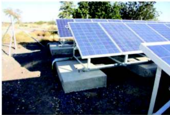
Figure 10. Example of solar panel installation (Alkantpan Village pilot study – Geotechnics Africa, 2010)
