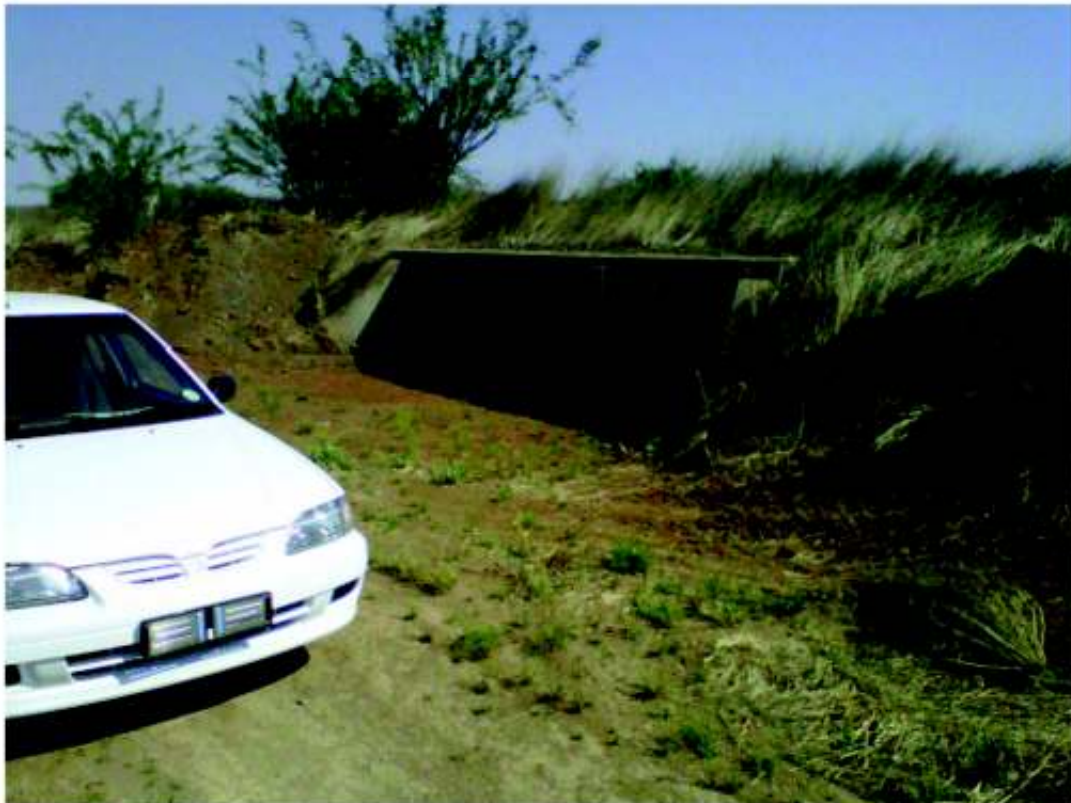
Figure 8. Existing Railway Culvert at south eastern corner of PV Site (approximately 2/ 1.8 x 1.2m)
