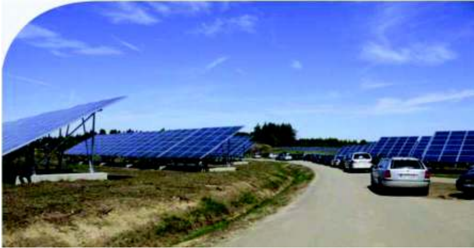
Photo 2 Illustration of foundations to be used per panel area with steel mounting brackets erected on them.
