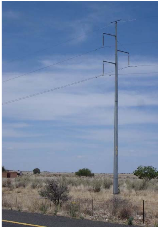
Plate 3.1: Photograph of a monopole steel tower similar to that which would be utilised for the proposed project (Photo: Reinhold Viljoen).
