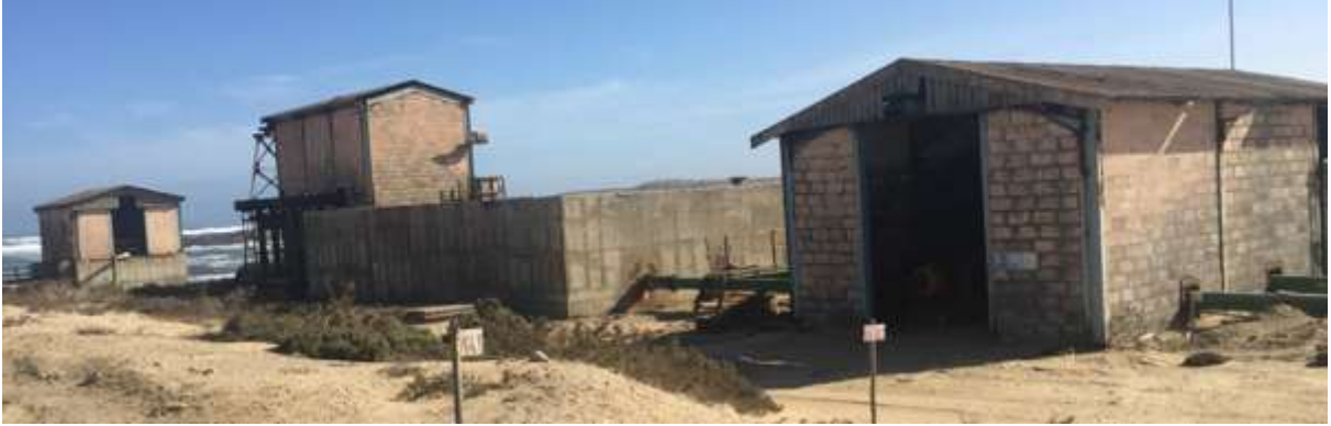
Tweepad Seawater Intake: Pump, crane & store building
