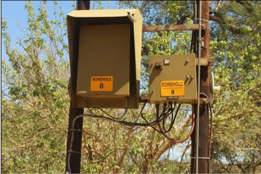
Figure 12: Borehole No:8 Switching station
