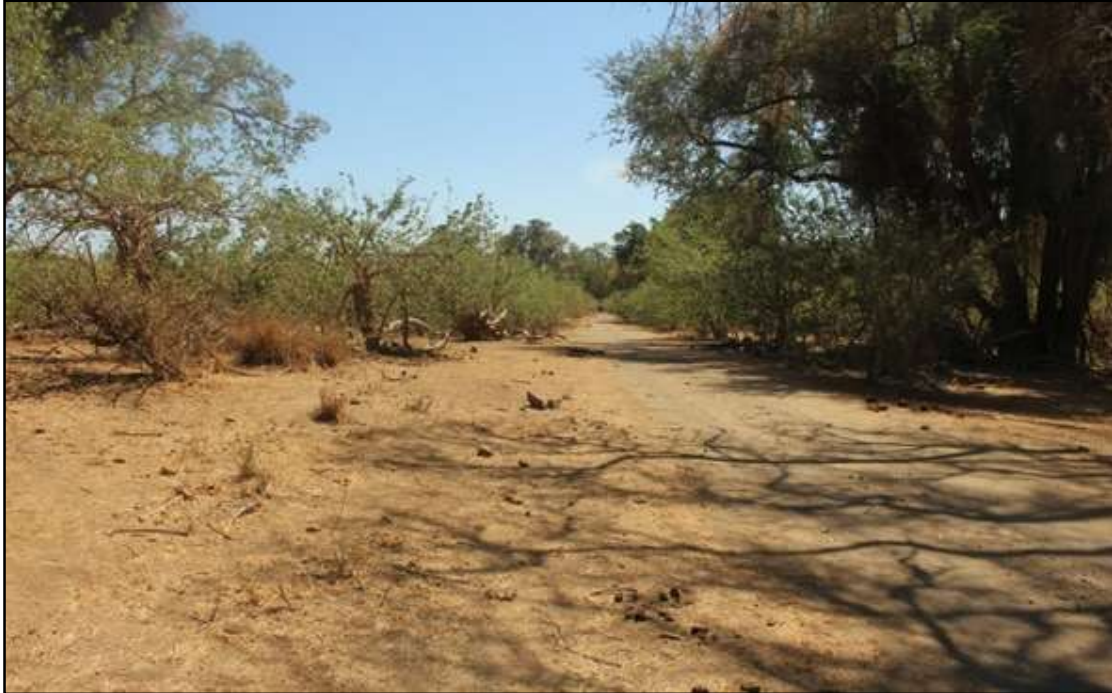
Figure 6: Main gravel access road that transverse alongside the powerline
