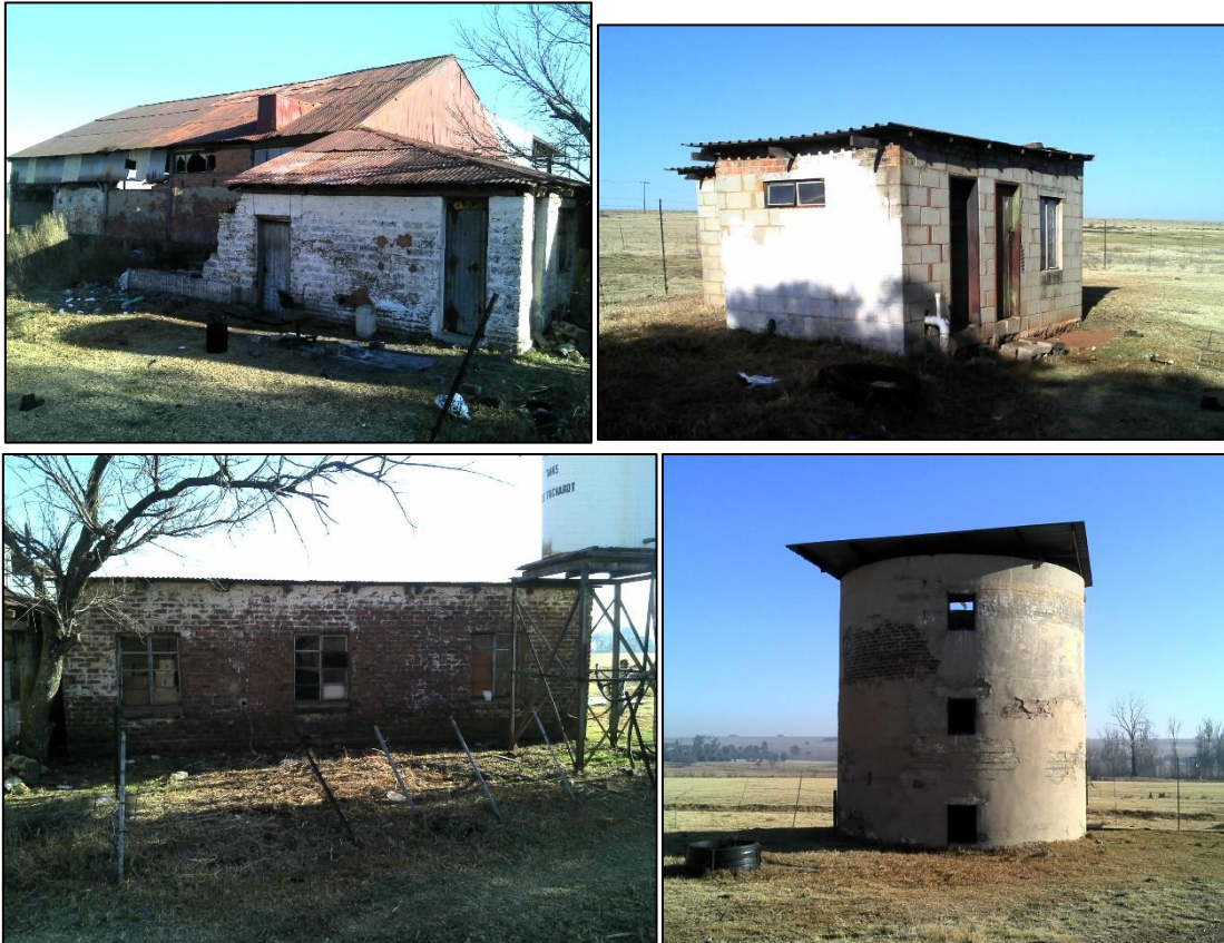
Figures 9 to 12: Buildings to the south of the R50 road. Only the large shed at upper left seems to have been present in 1945.
