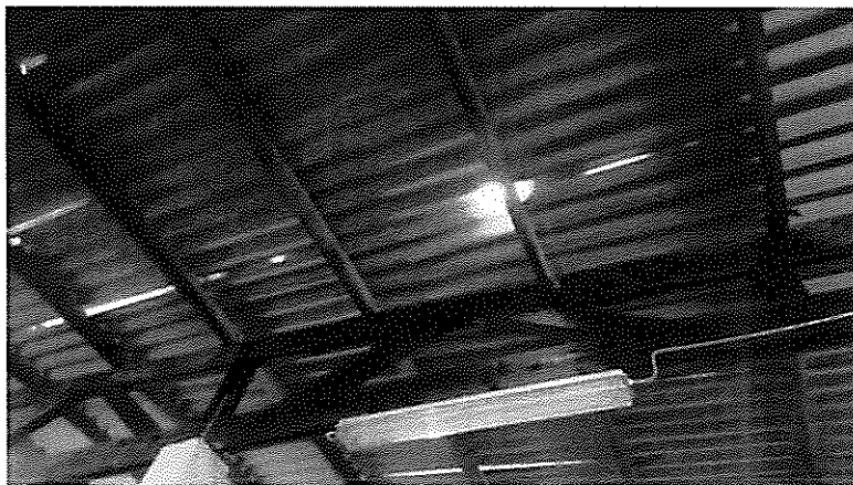
Figure 5-14 Openings through roofsheets
