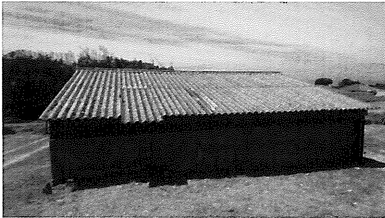
Figure 5-13 Existing roofsheets of seawater reservoir
