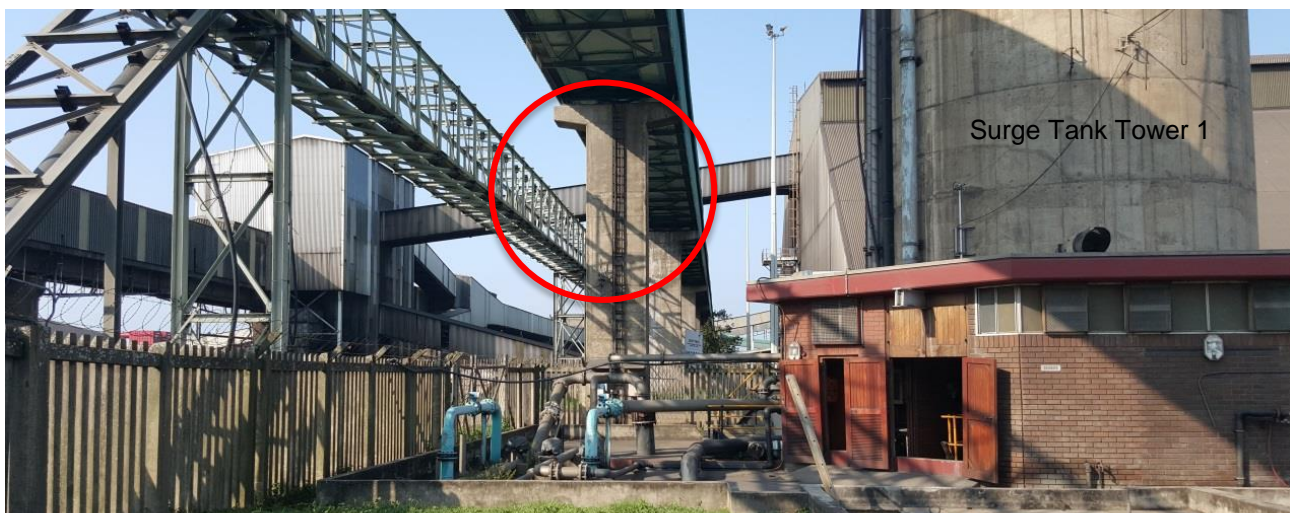
Figure 3: Hillside take-off point from Foskor seawater pipeline to a connection supported on existing conveyor 07 concrete trestle next to the Mhlathuze Surge Tank Tower 1.
