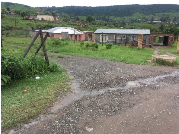
Fig. 3 END OF KHAMBULE ROAD (CONSTRUCTION)
