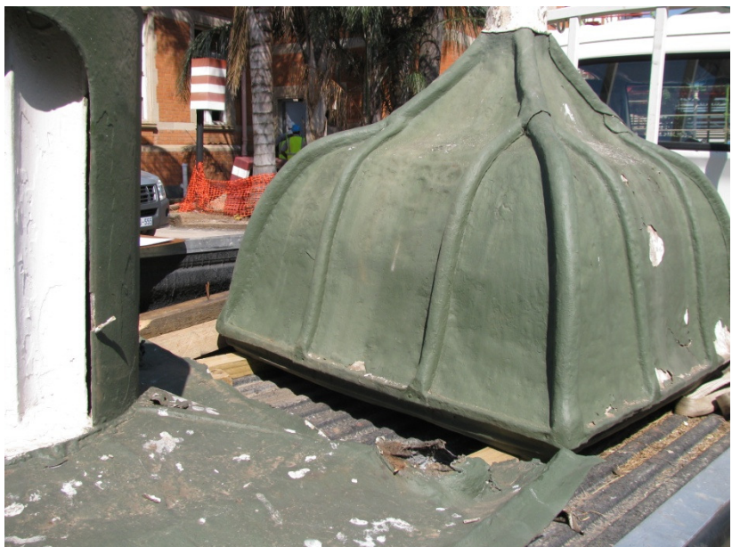
Domed roof and ventilator in Foreground.
