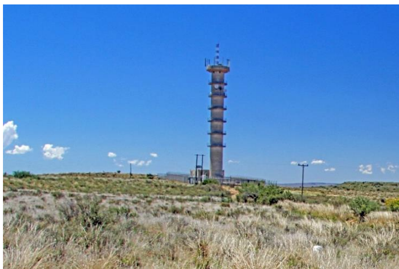
Figure 10: The proposed development site already also houses a microwave tower on the western side of the site.
