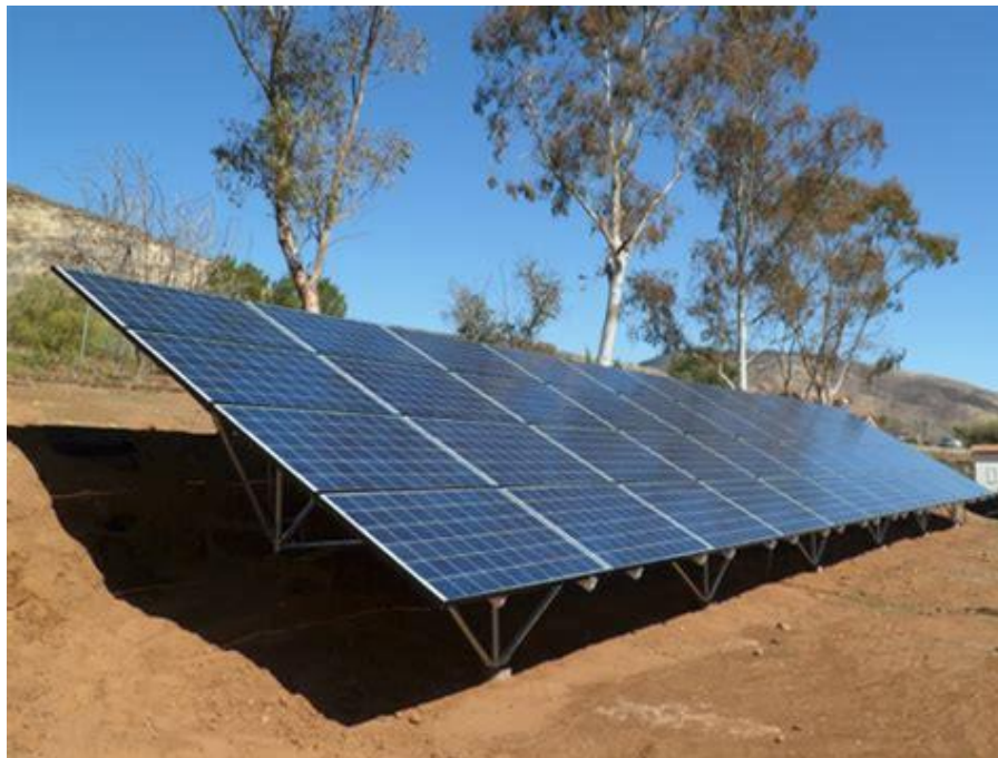
Figure 14: A fixed or rack structure PV solar mounting
