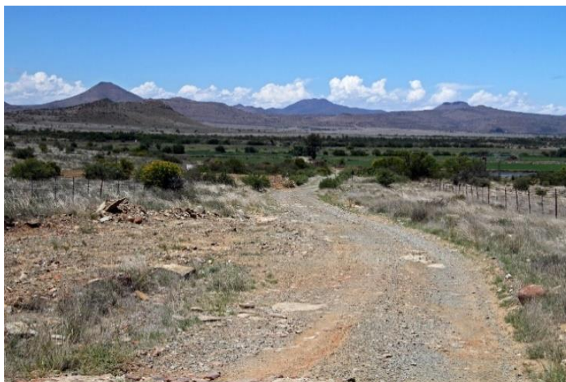
Figure 7: The gravel road from the N10 to the Knutsford siding, from which will be the access road to the proposed development site.
