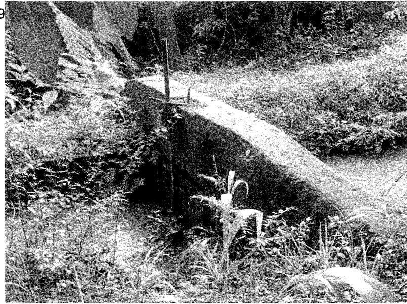
Figure 30: Photo of sluice gate(see map Figure 24).
