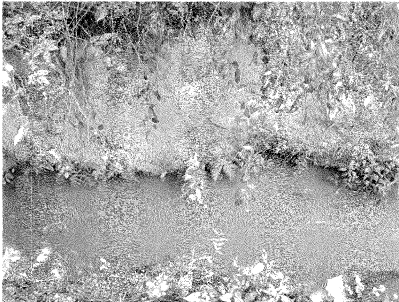
Figure 31: Canal flowing from weir.
