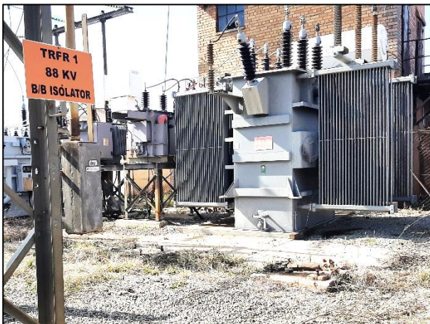
Images 4: Venterdorp Munic 88/11kV 2x 10MVA substation
