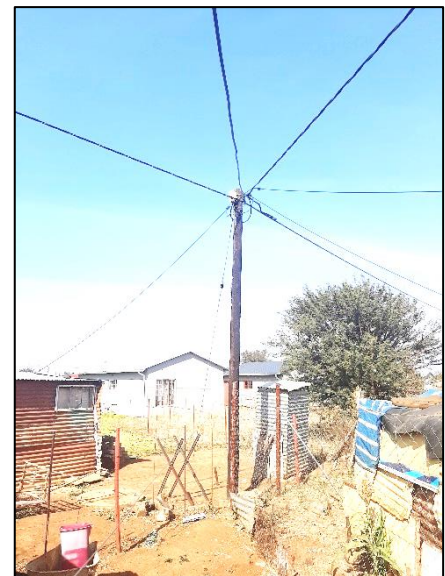
Images 7: Existing Low Voltage Aerial Bundled Conductor & Airdac reticulation networks
