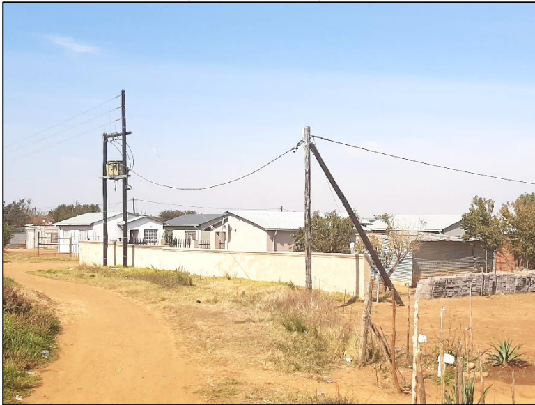
Images 5: Typical platform mounted, 11kV/231V transformers
