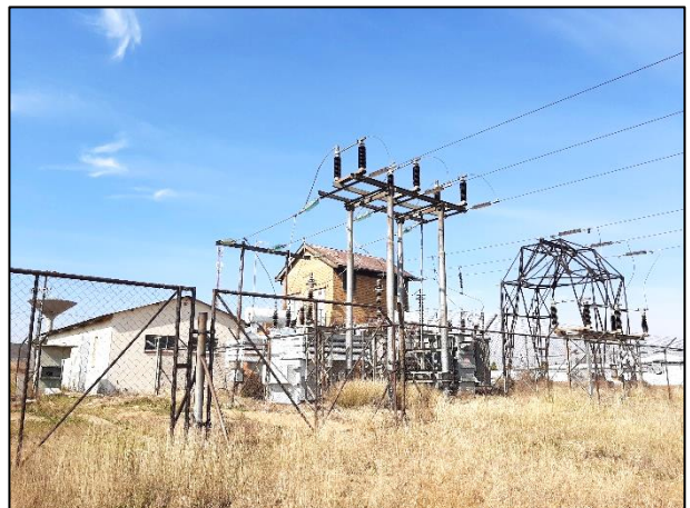
Images 4: Venterdorp Munic 88/11kV 2x 10MVA substation
