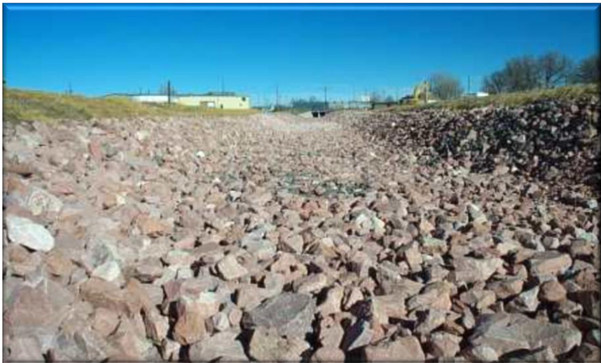
Figure 3-2 Image of a typical rip rap armoured channel (HEES, 2022)
