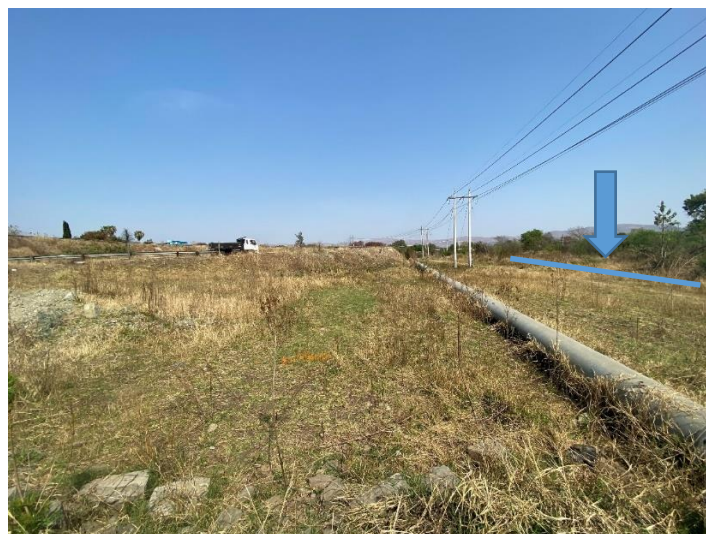
Figure 3-6 Existing maintenance roads (shown with blue arrow)
