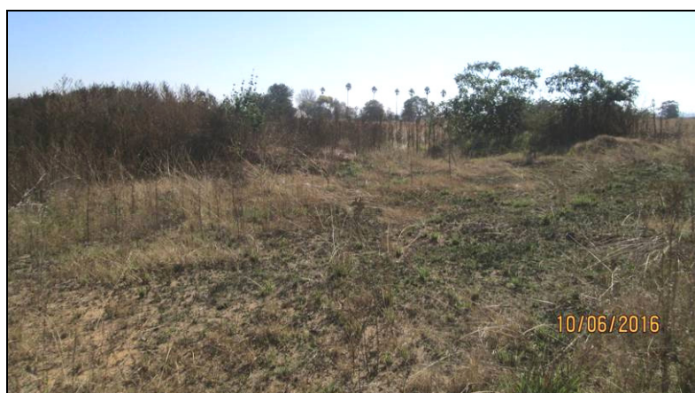
Photo 5.8: A view of Geotechnical Zone PQ, where excavations took place and spoil was dumped.
