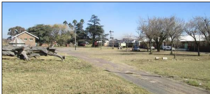
Photo 5.7: A view of the Transnet Railway Station and offices
