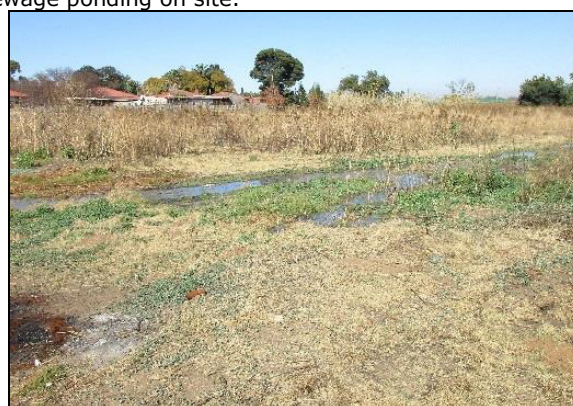
Photo 5.16: A view of the artificially wet area east of the site due to leaking sewage.
