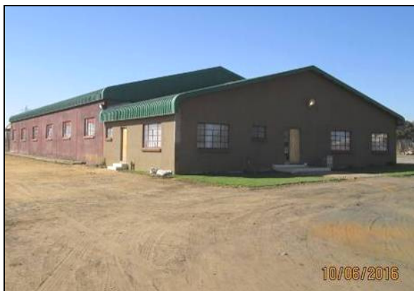
Photo 5.1: The church (Apostolic Mission Revival) located in the southern corner of the site.
