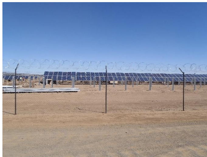
Figure A.6. Example of PV Technology (DFFE, 2019)
