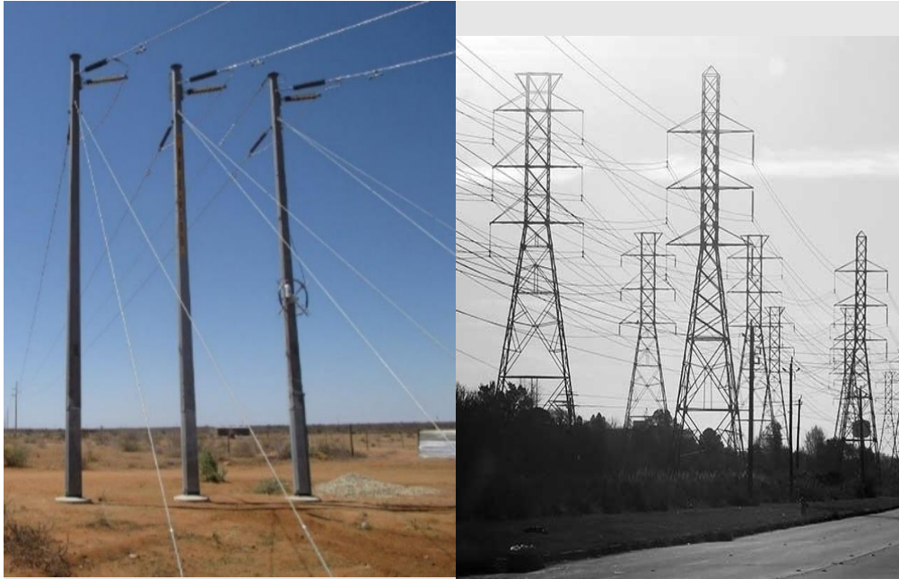
Figure 4-2: Typical 132kV monopole type (left) or lattice-type pylons (right) design
