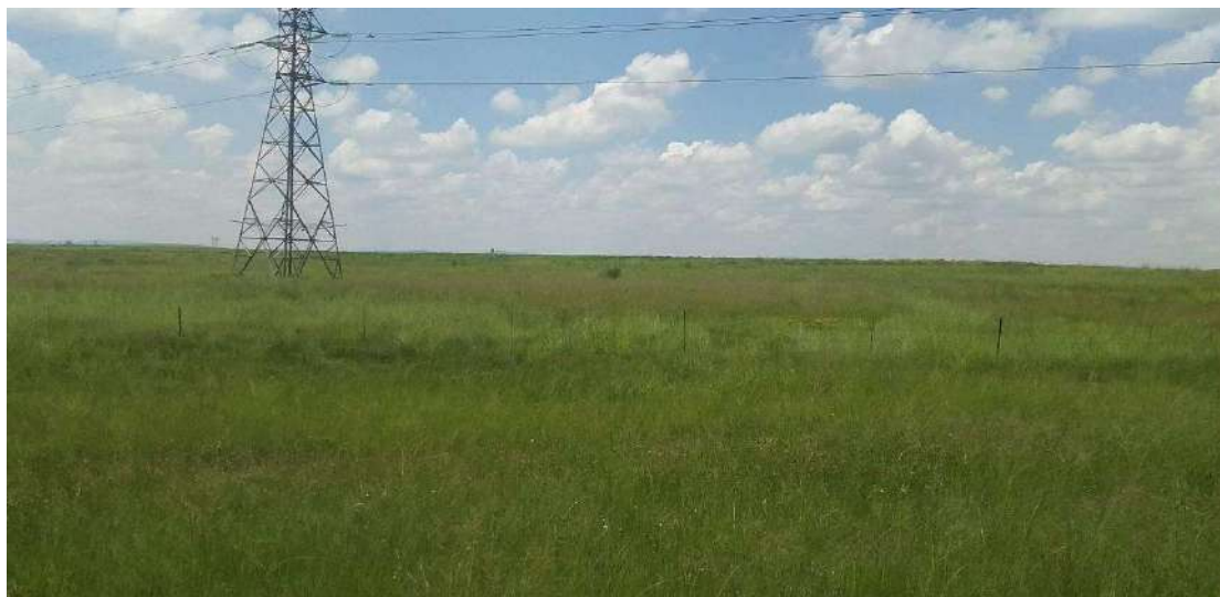
Figure 51: Infrastructures (Electrical Power lines) within the proposed project area. (
