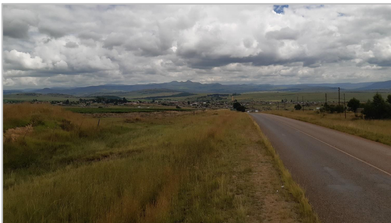
Figure 27: R543 from eMkhondo to Dirkiesdorp (Photograph by SC, 2022)
