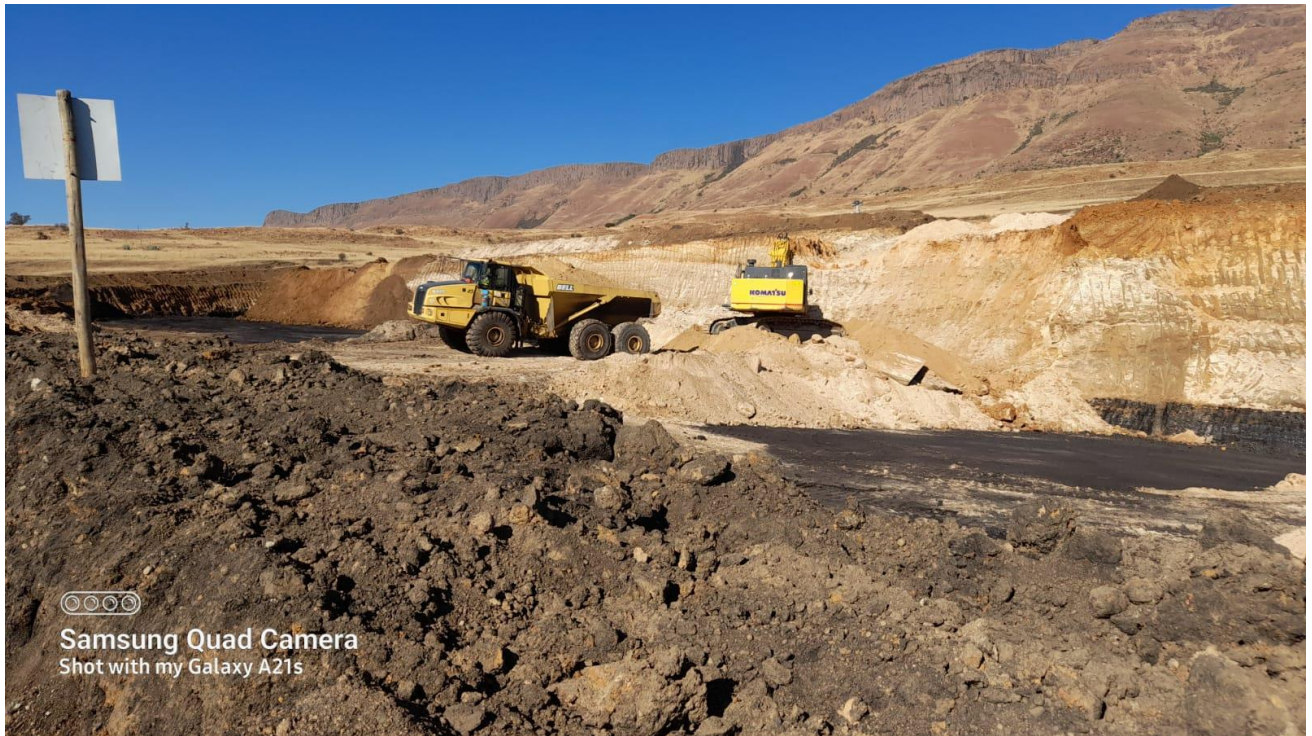
Figure 6: Typical example of open cast operation
