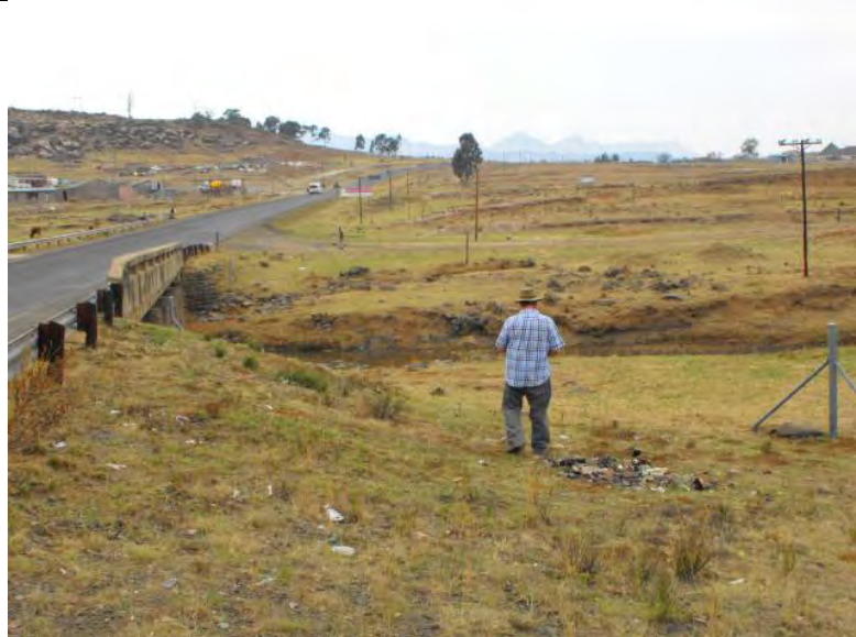
Figure 11: View of the Phase 2 pipeline along the eastern split. The pipeline will be installed adjacent to the road. The pipeline will cross the seasonal stream by means of a bridge attachment and the stream will therefore not be affected.
