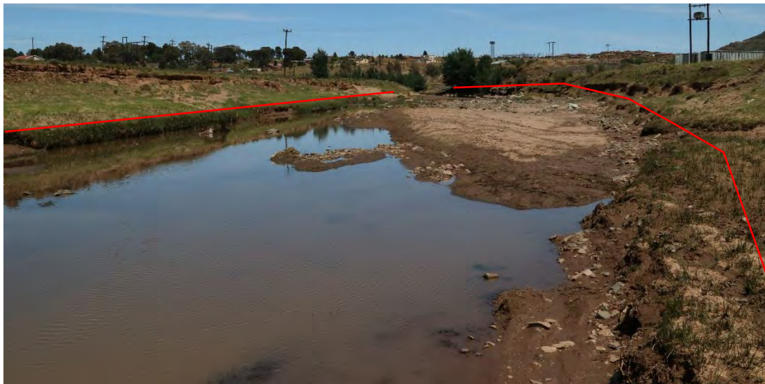
Figure 9: View of the marginal (red). Note again erosion with sparse vegetation.
