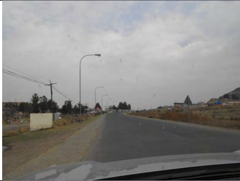
Figure 10: View of the Phase 2 pipeline along the eastern split. The pipeline will be installed adjacent to the road.
