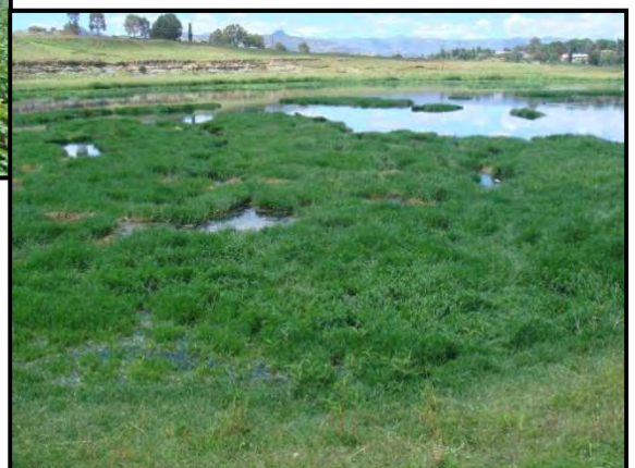
Figure 12: Overgrow in oxidation pond
