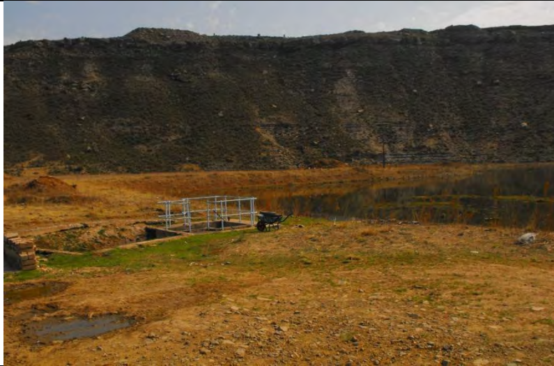
Figure 1: View of the site as seen toward the north. Note the existing oxidation ponds and the mountainous terrain in the background.
