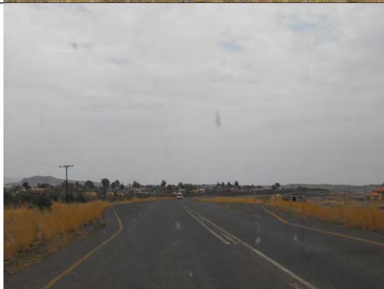
Figure 12: View of the Phase 2 pipeline along the western split. The pipeline will be installed adjacent to the road.
