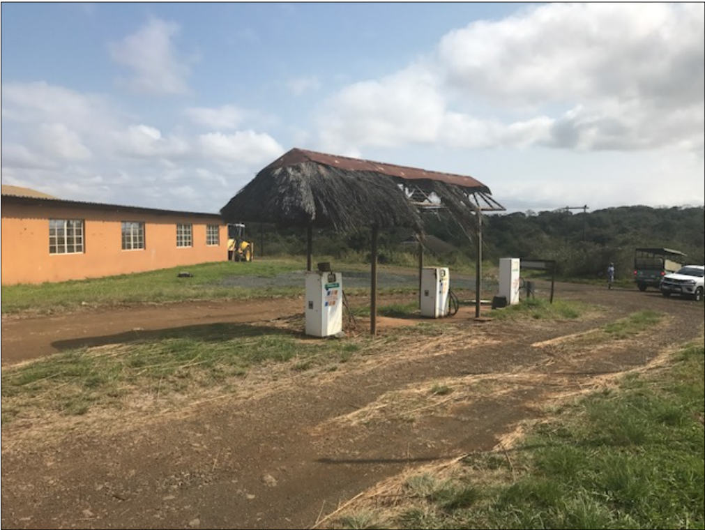
Photo 1: View of pumps.
