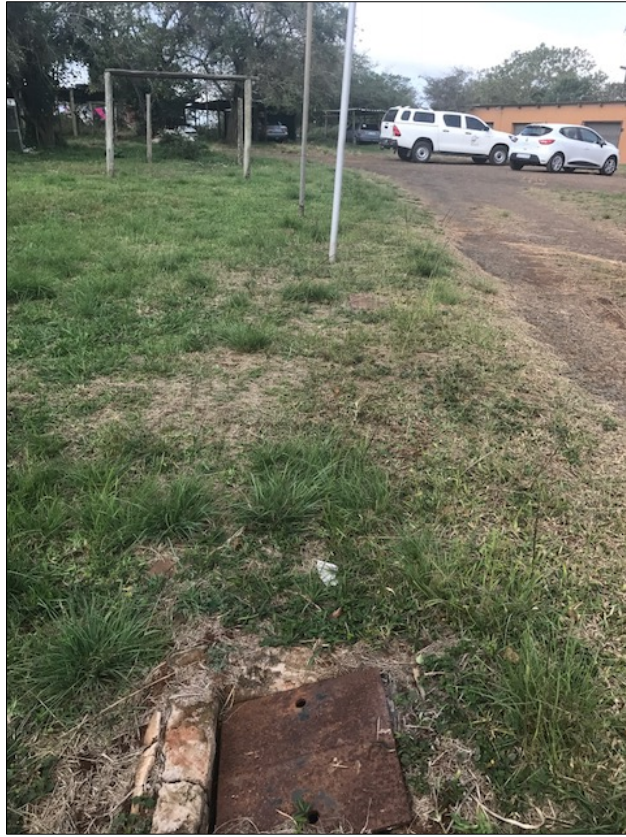
Photo 5: Tank manhole 3 and vent
