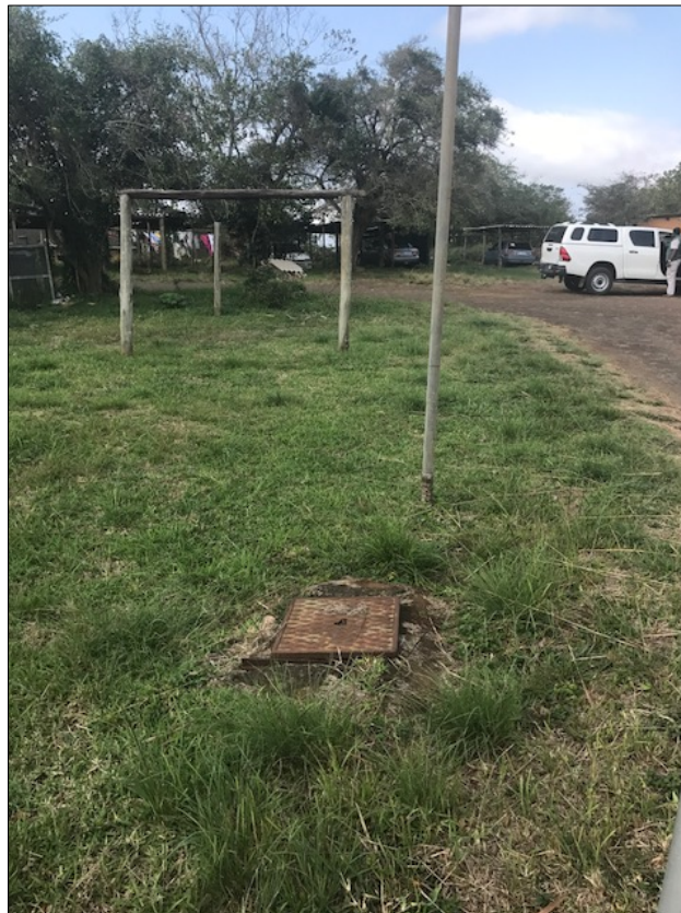
Photo 4: Tank manhole 1 and vent
