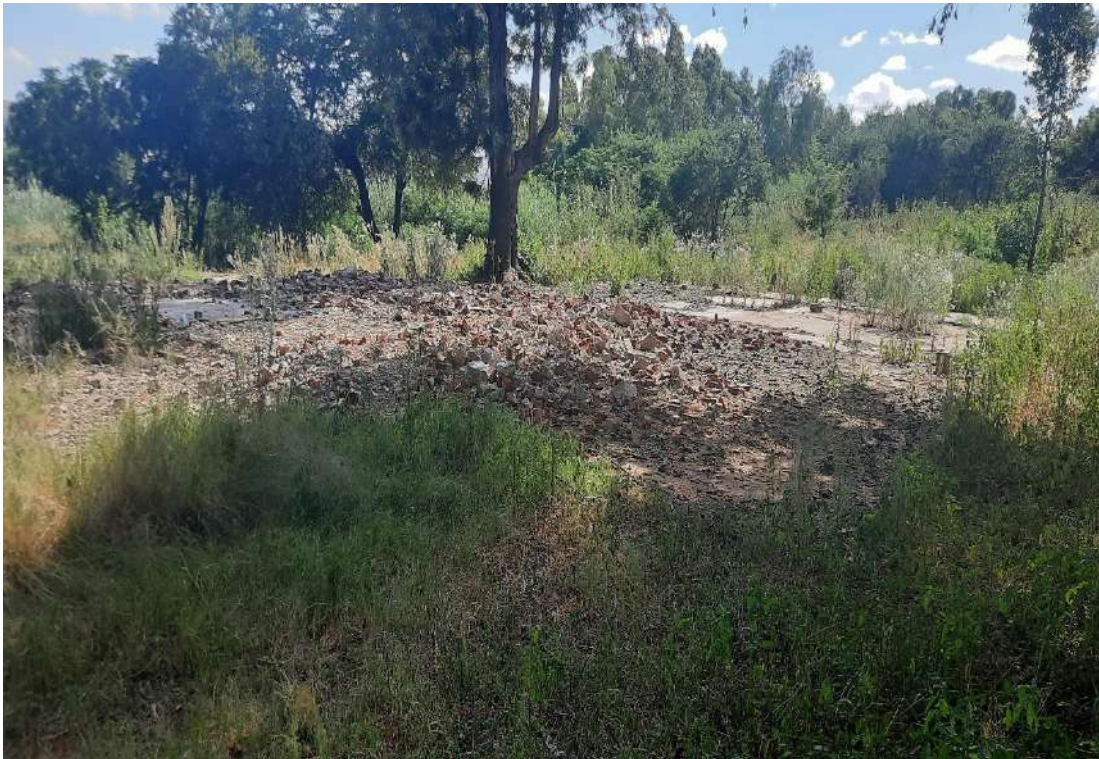
Figure 13: The foundations of another recent structure/homestead in the area.
