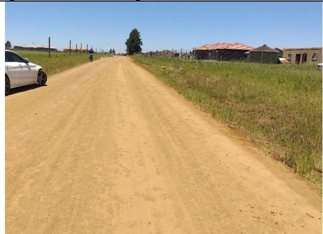
Photo 16: A view from the existing access gravel road heading south towards Madadeni Road (P483)
