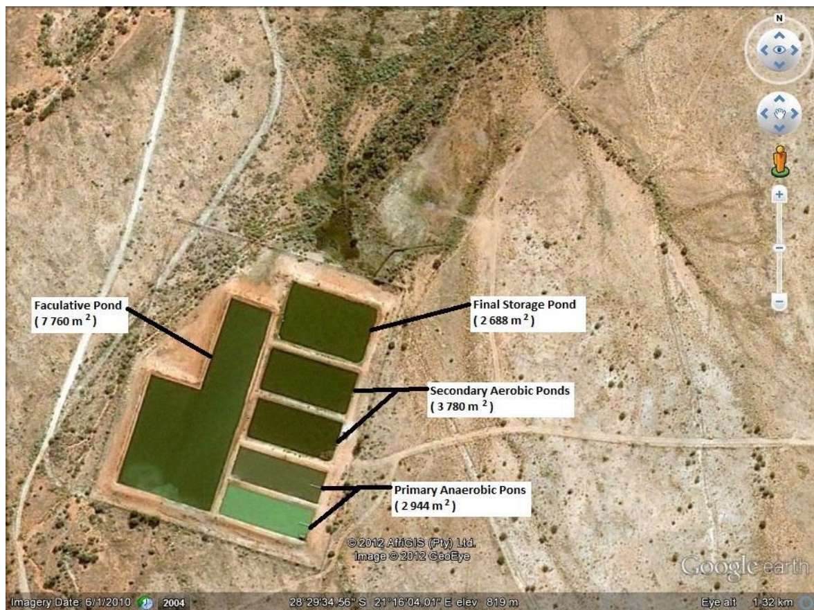
Figure 2: Current layout of the existing oxidation pond system at Louisvale Rd
