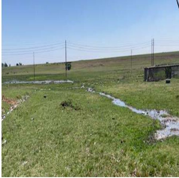
Powerline Route 2a
