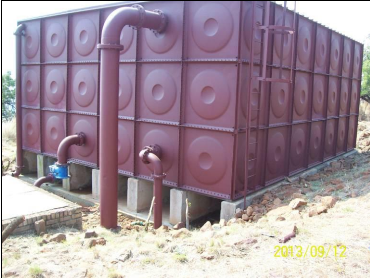
Figure 2: The existing 200 m 3 Tierkloof Reservoir
