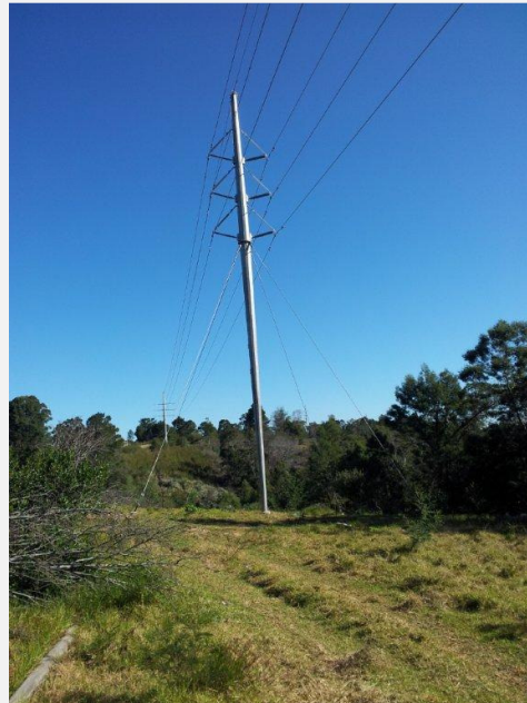
Figure 5: Guyed suspension Tower
