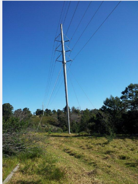
Figure 5: Guyed suspension Tower
