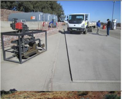
Photograph taken from the centre of the site towards the south west. Take note of the drainage channel that has been installed for the collection of dirty stormwater. The drainage channel feeds into an oil separator where the dirty oil is separated into a hazardous waste container.
