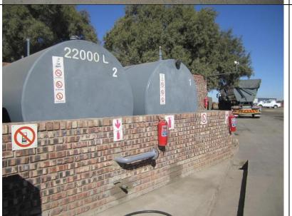
Photograph taken from the centre of the site towards the south of south west. Visible are the existing storage tanks used for the storage of diesel. Notice the bunded wall and appropriate signage and equipment is in place.
