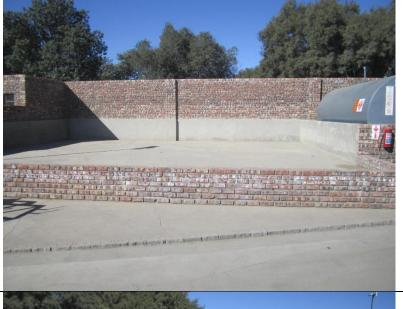
Photograph taken from the centre of the site towards the south. Visible is the proposed site for the new storage tanks. Notice the existing storage tanks on the right that is separated by a wall.
