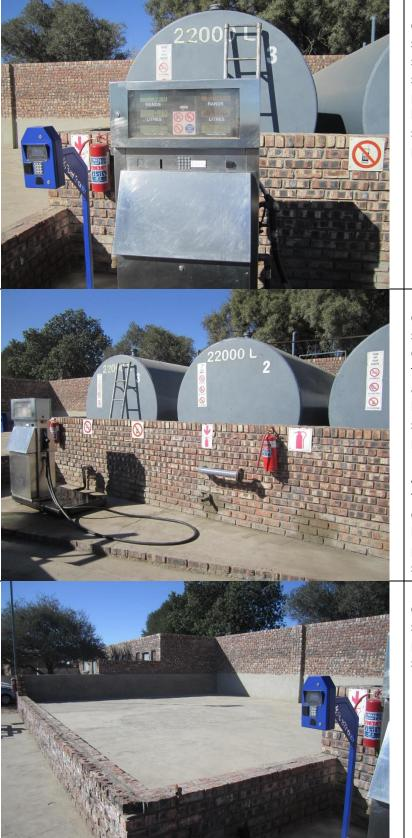
Photograph taken from the centre of the site towards the south. Visible are the existing storage tanks used for the storage of diesel as well as a pump station. Notice the bunded wall and appropriate signage and equipment is in place.
