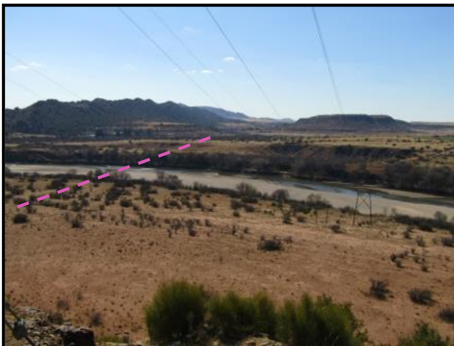
Photo 5: Proposed crossing over the Orange River to the left of the existing 66kV
