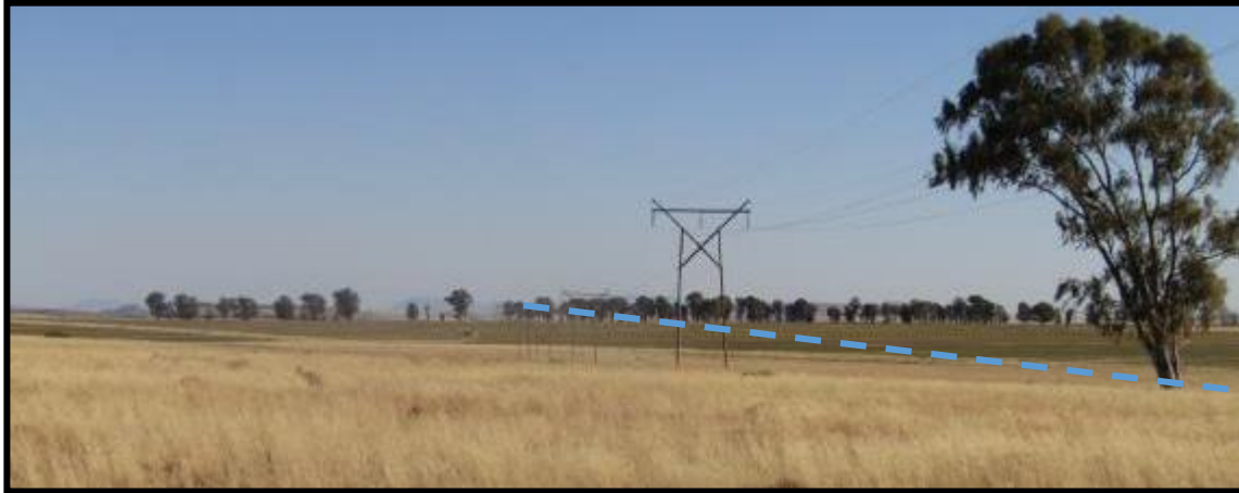
Photo 9: Southern view of the Proposed Powerline along the 66kV Line across cultivated lands
