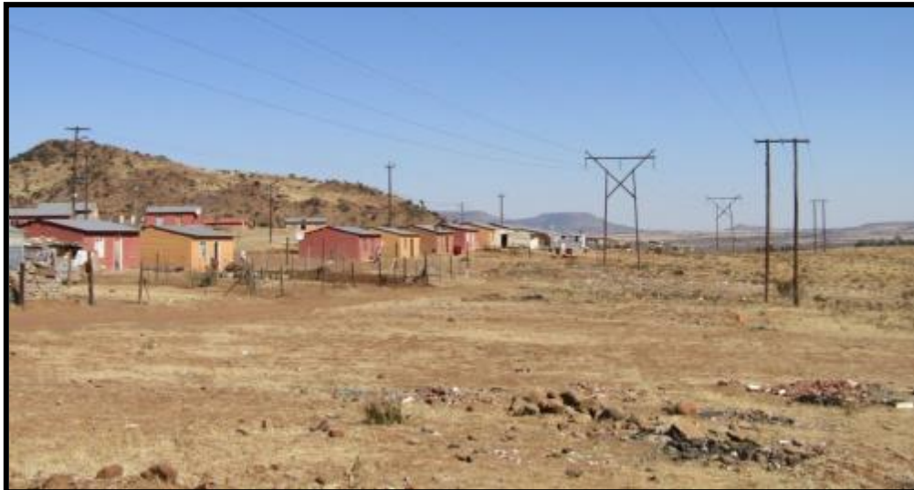
Photo 3: View of the existing power-lines in the vicinity of Area 13, Dukathole
