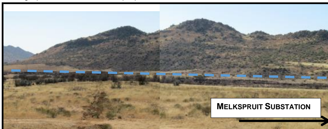
Photo 1: Proposed route along the ridge next to the existing 66kV Powerline
