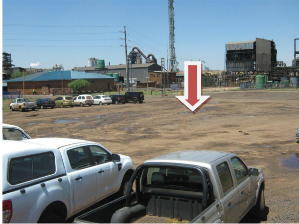
The proposed substation will be located on the vacant land on the left of the Rhovan Mine entrance gate
