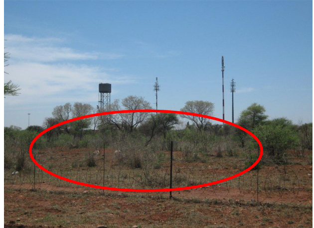
Substation Alternative will be located to the south of Bethanie village
