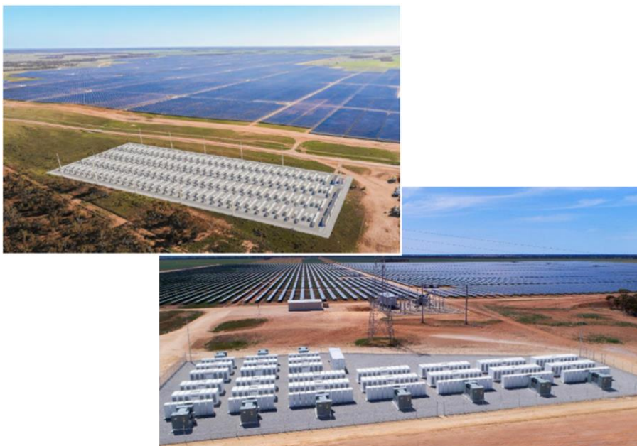
Figure 16: Images of typical centralized AC coupled BESS systems servicing solar power farms
