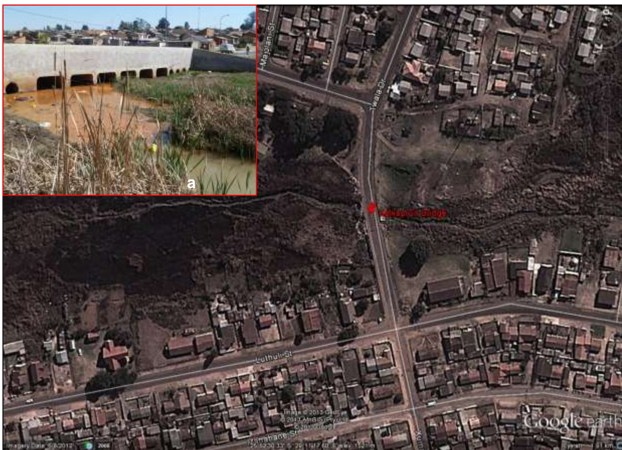
Figure 4: Aerial map showing the location of the Kalkspruit bridge, (a) picture of the existing structure
