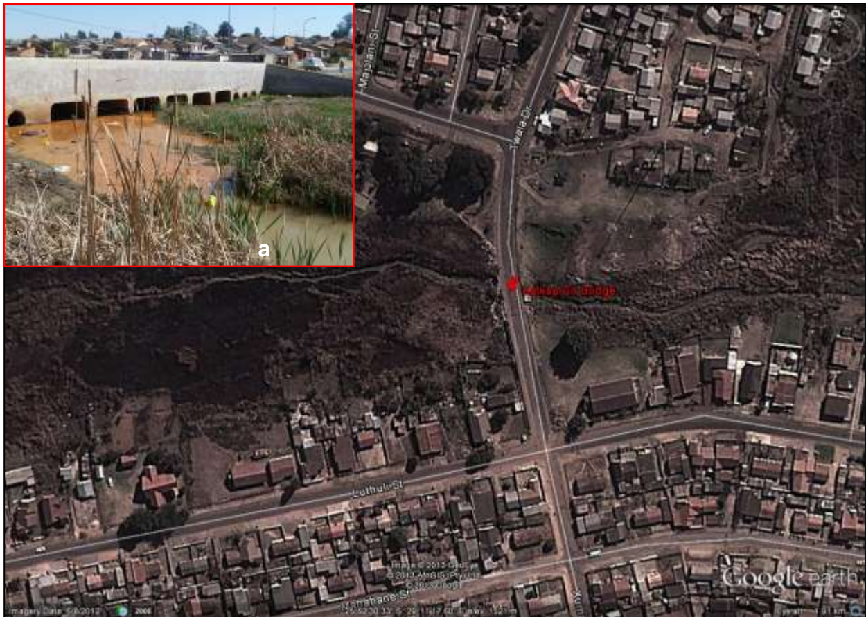
Figure 1: Aerial map showing the location of the Kalkspruit bridge, (a) picture of the existing structure
