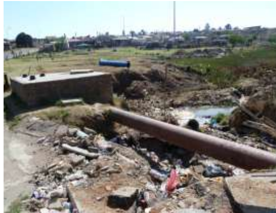
Figure 3: Excessive illegal dumping.
