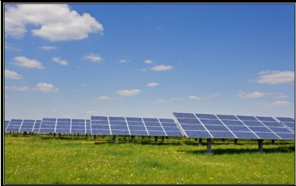
Figure 3: Example: Vegetation growing underneath the panels for stabilisation of the soil.
