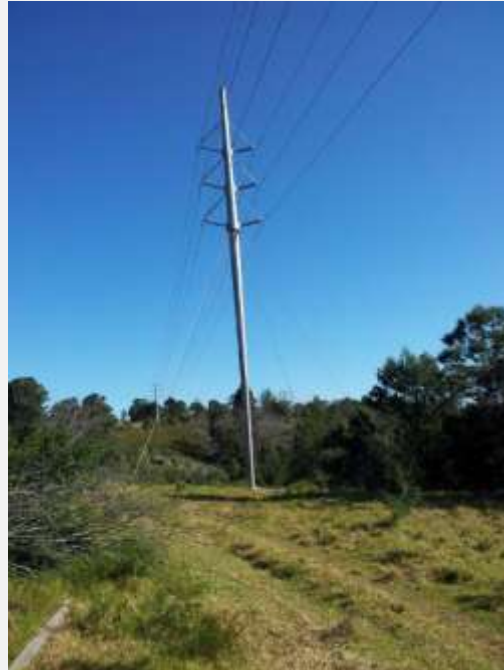
Figure 3: Guyed suspension Tower
