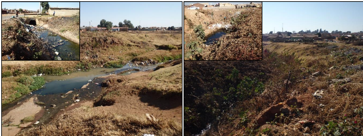
Figure 9: Several large stormwater channels were identified draining into the river channel. Left: A formalized stormwater channel drains water from Freedom Street into the river. Note that at the outlet, the concrete base has been under scoured. Right: A large informal stormwater channel is located within the south-western portion of the study area (from Polaris Street).
