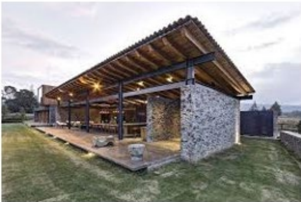
MONO PITCH ROOF WITH LARGE ROOF OVERHANG
