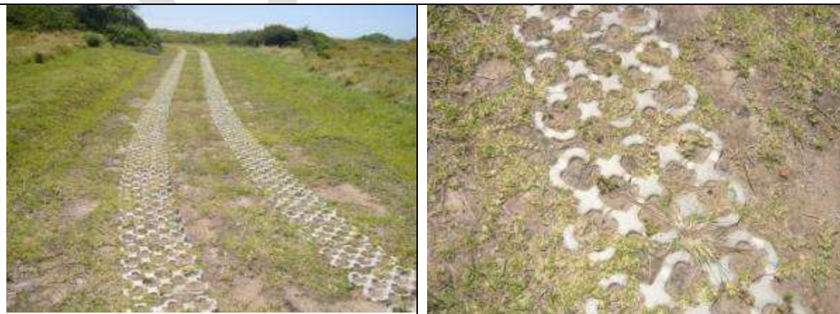
Figure 5-1: Proposed internal road structure
