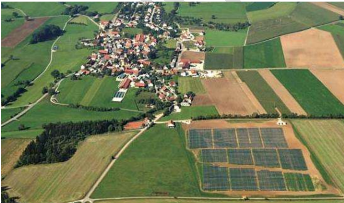
Figure 1-9: Example of a solar PV facility consisting of 12 arrays. similar size to the 10 MW facility proposed for Peddie
